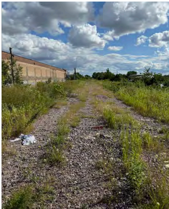
Current condition of trail at Armitage Avenue looking south.
